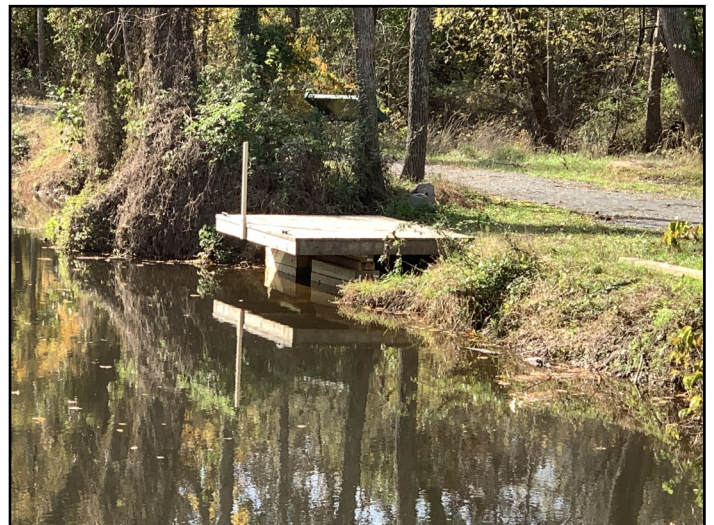
Griggstown dock completed
