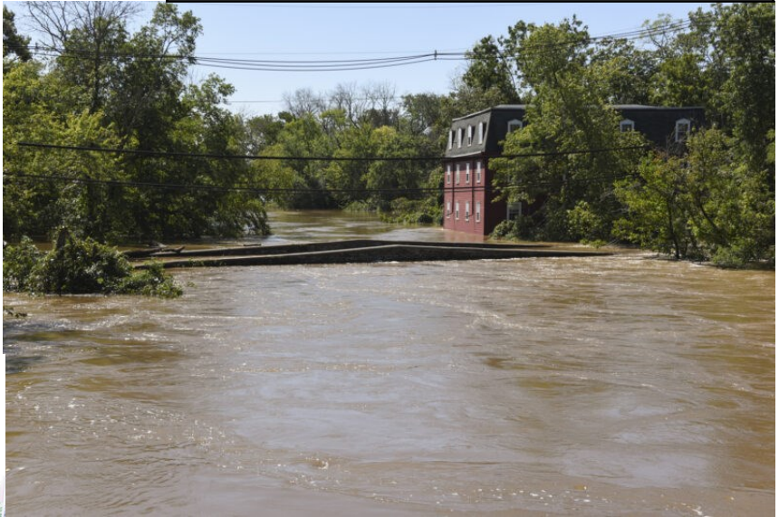
The Kingston Mill withstood the flooding remarkably well because of the way the owners restored it after the last flood. While a trace of water did get onto the first floor, the design of the floor and wallboards make the mill resilient. The owners also used their elevator to move items from the first to second floor. (Photo: courtesy of Town Topics)
