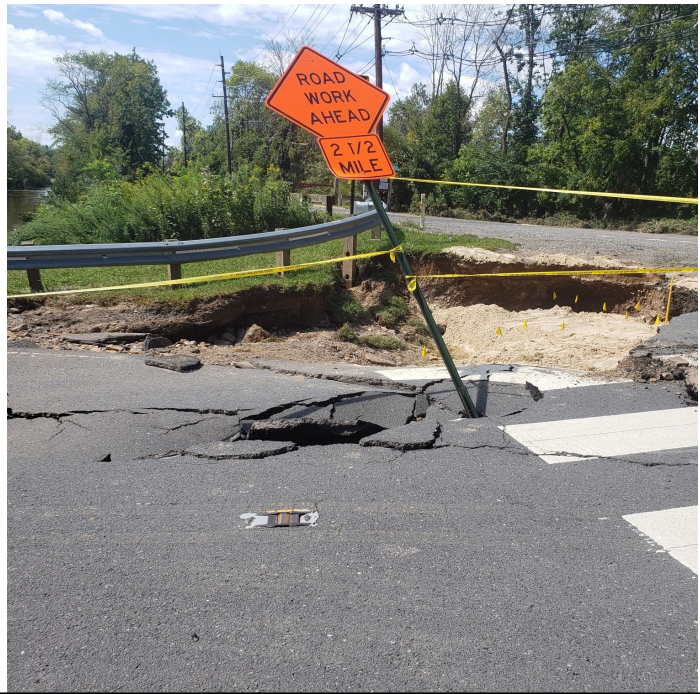
A sinkhole on Quakerbridge Road near the canal in Port Mercer Photo by Patricia Kallesser.
